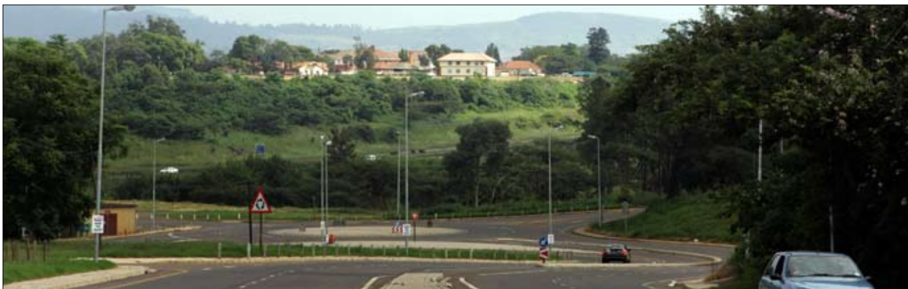
Changing the face of Pietermaritzburg: the new Senior Boarding block as seen from across the valley in Hesketh Drive, Hayfields
